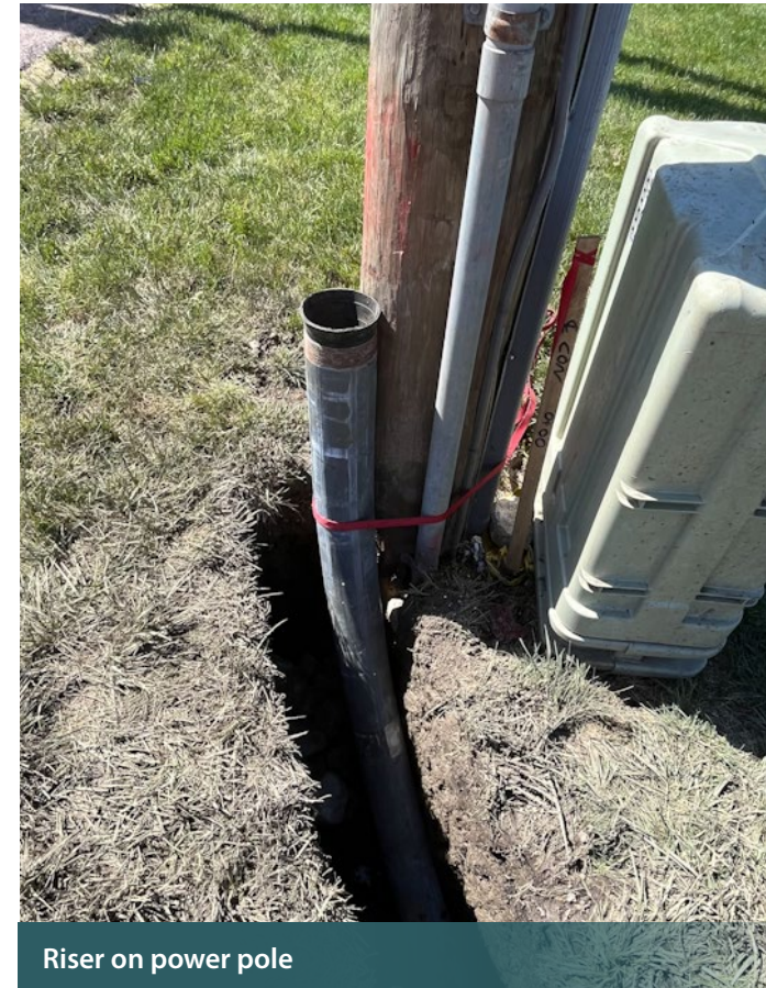
Splice box ready for backfill
