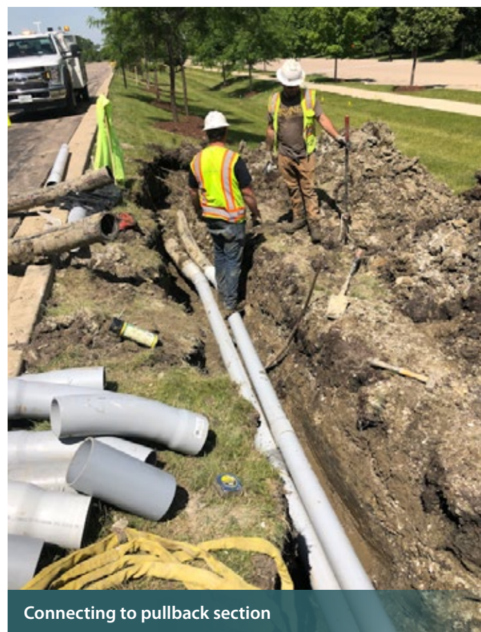
Conduit connection in trench box
